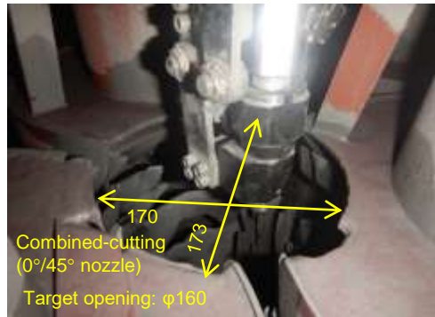
(c) Steam separator (triple cylinder center)
