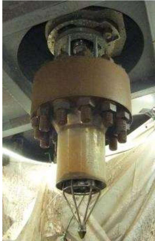
Removal of fragments of the (upper) RPV nozzle
